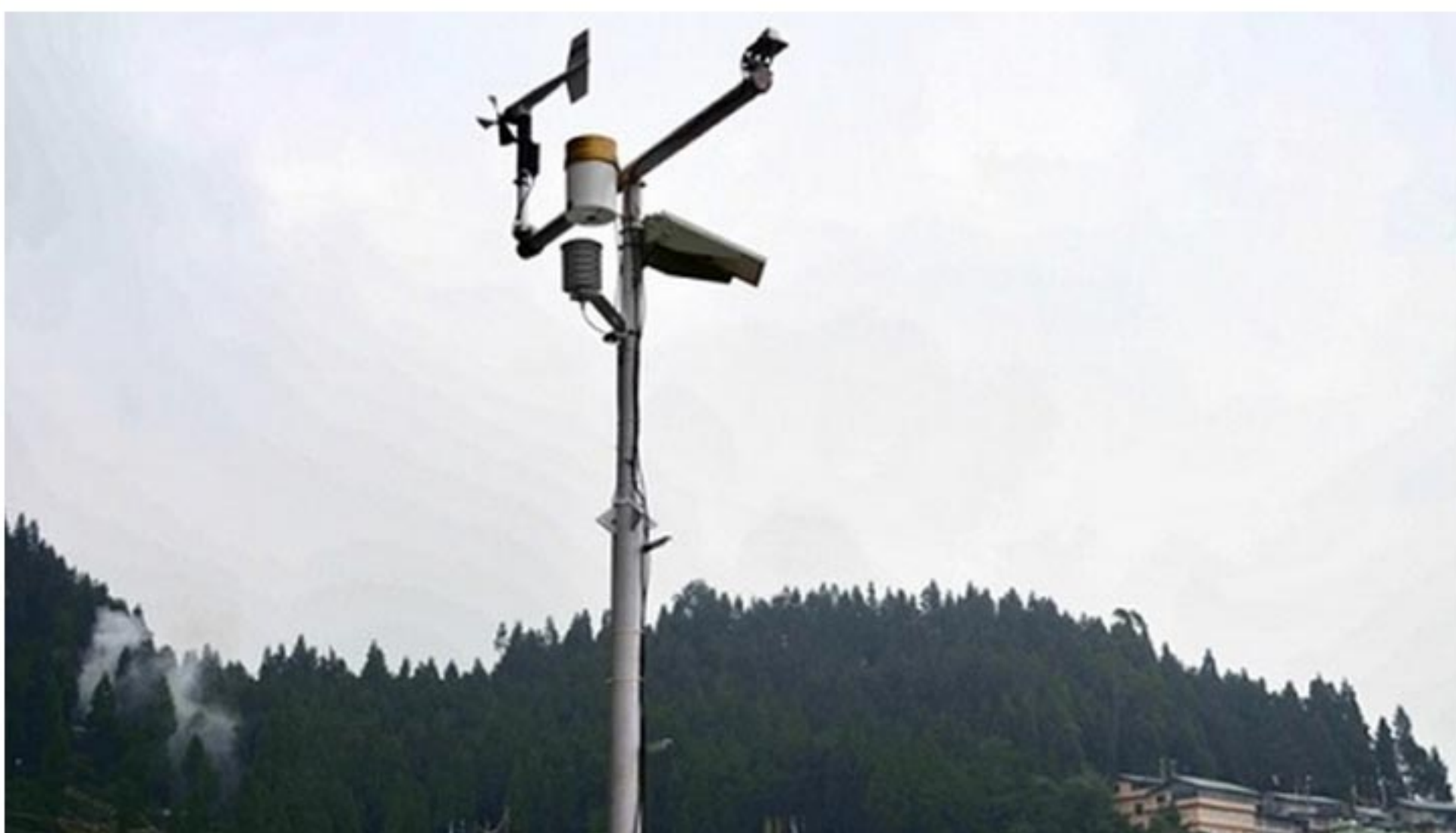
Sensors at Chandmari Village in Sikkim's Gangtok District. Image: India Science Wire
