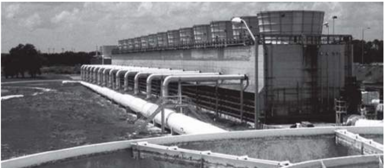
Figure 2-3. Cooling Tower
