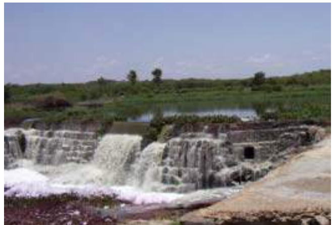
Hyderabad, India – wastewater being diverted over weir into irrigation canals. Source: International Water Management Institute
