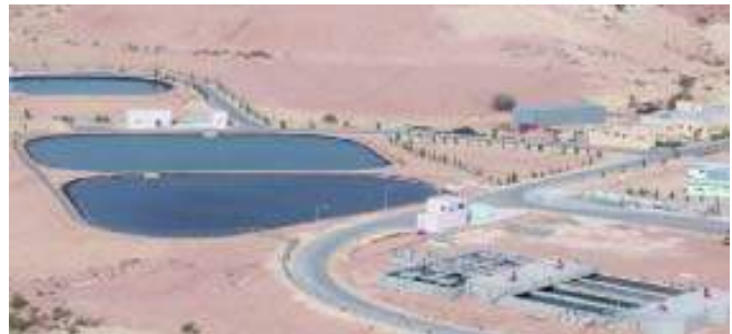
Wadi Musa secondary treatment plant and storage ponds serving communities in the vicinity of Petra, Jordan. Photo courtesy of Bahman Sheikh
